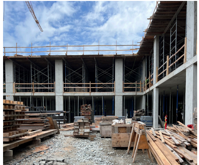
Photo: hcma architecture + design | WHM Structural Engineers
