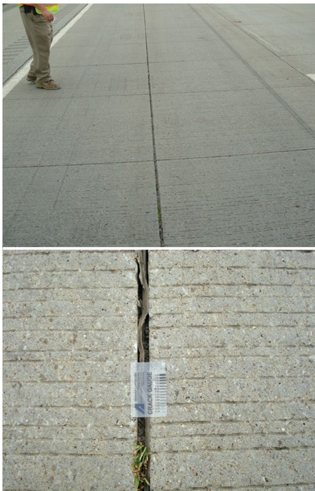
Figure A.5. COA-B overlay with tied lane joints and untied mid-lane longitudinal joint after eight years of service
