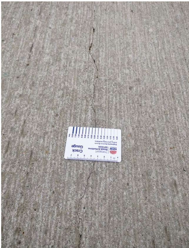
Figure 6.1. Reflective cracking in an overlay without fibers (top) and in an overlay containing macrofibers (bottom)
