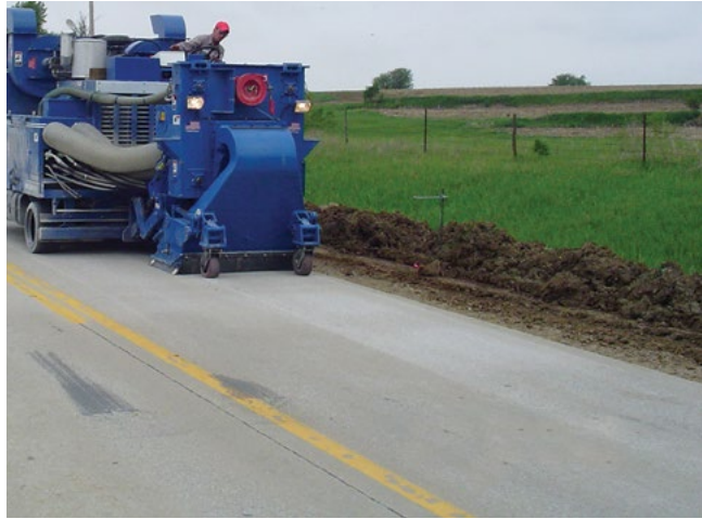
Figure C.6. Shotblasting of a concrete surface
