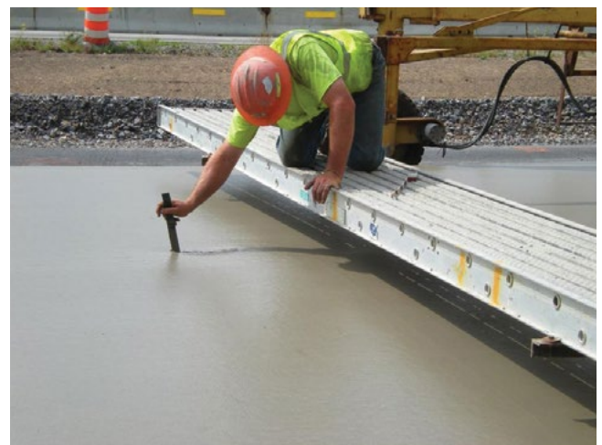
Figure 8.10. Manual verification of dowel placement
