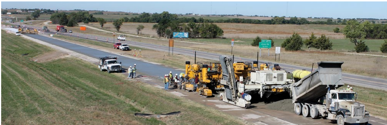
Figure C.8. Placement of a thin COC-B overlay
