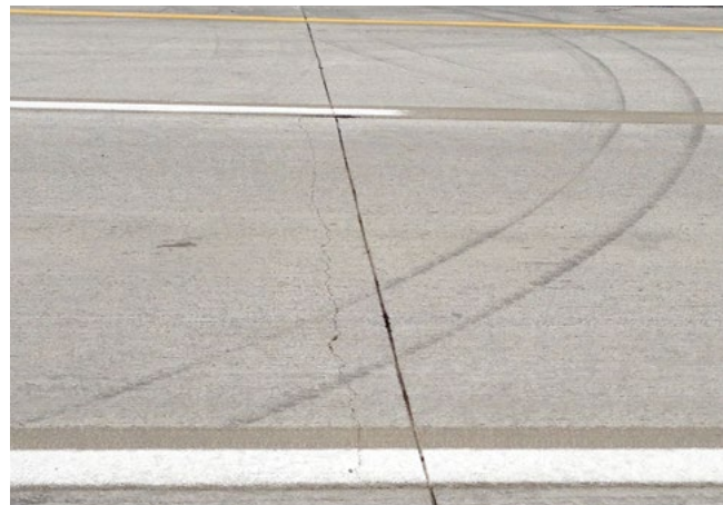
Figure A.7. Double-crack resulting from failure to match the sawcut with the underlying joint location in a COC–B overlay
