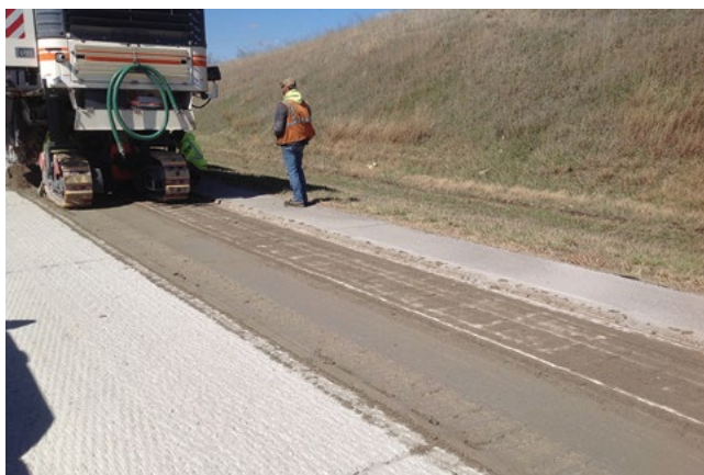
Figure 8.14. Typical concrete pavement milling operation in progress
