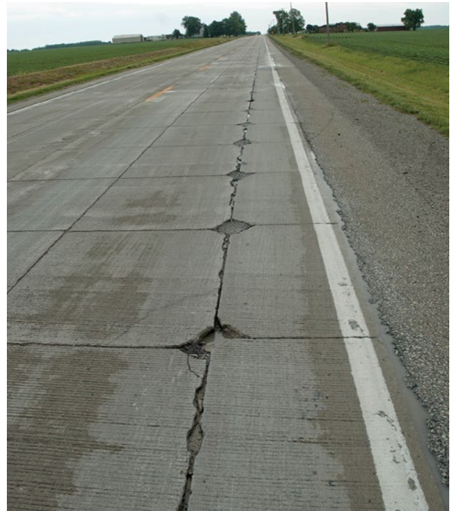
Figure A.3. Concrete overlay on composite pavement photographed in 2012 after 13 years in service, with the overlay exhibiting interior corner deterioration due to longitudinal joints in the wheel paths
