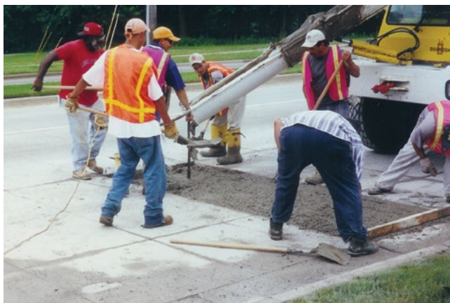
Figure 8.13. Finishing and curing of a concrete overlay repair
