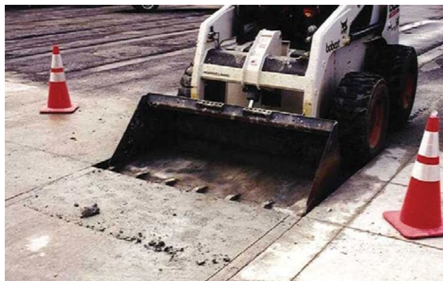
Figure 8.12. Removal of overlay panels
