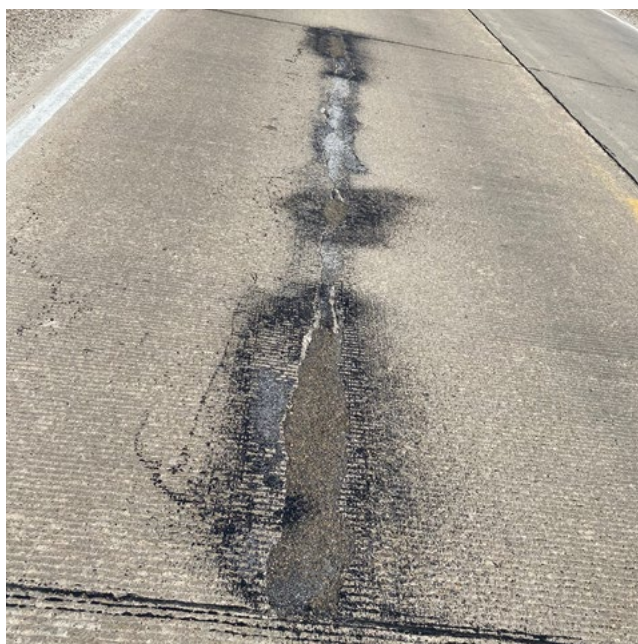
Figure C.2. Deteriorated longitudinal crack in a COC–B overlay
