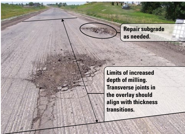
Figure 8.4. Area where the milling and concrete overlay depths are to be adjusted to address isolated locations where the remaining pavement depth is inadequate
