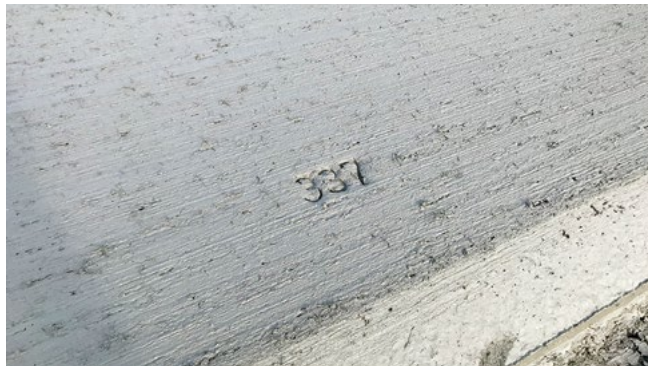
Figure 6.4. Surface texture of concrete overlay with synthetic macrofibers
