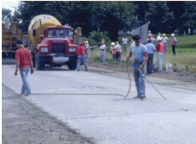
Figure C.7. Use of compressed air to clean existing concrete in front of the paver
