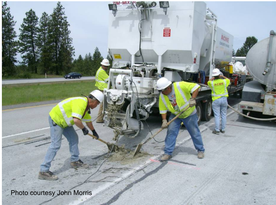
Figure 62 Placement of patching material.
