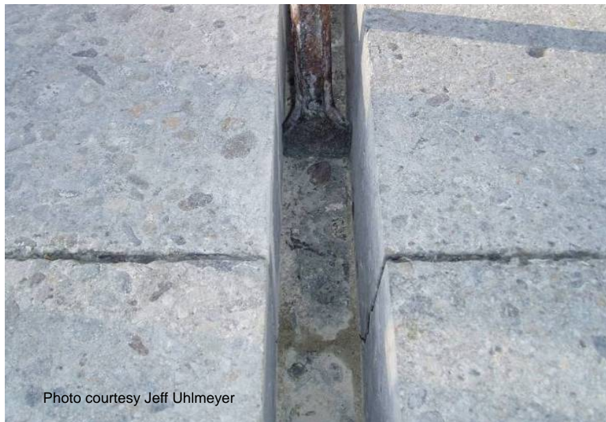
Figure 25 Leveling the bottom of the dowel bar slot.
