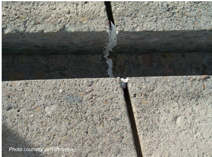
Figure 50 Caulked dowel bar slot.
