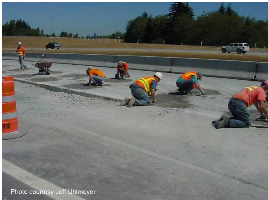
Figure 71 Finishing patching material.
