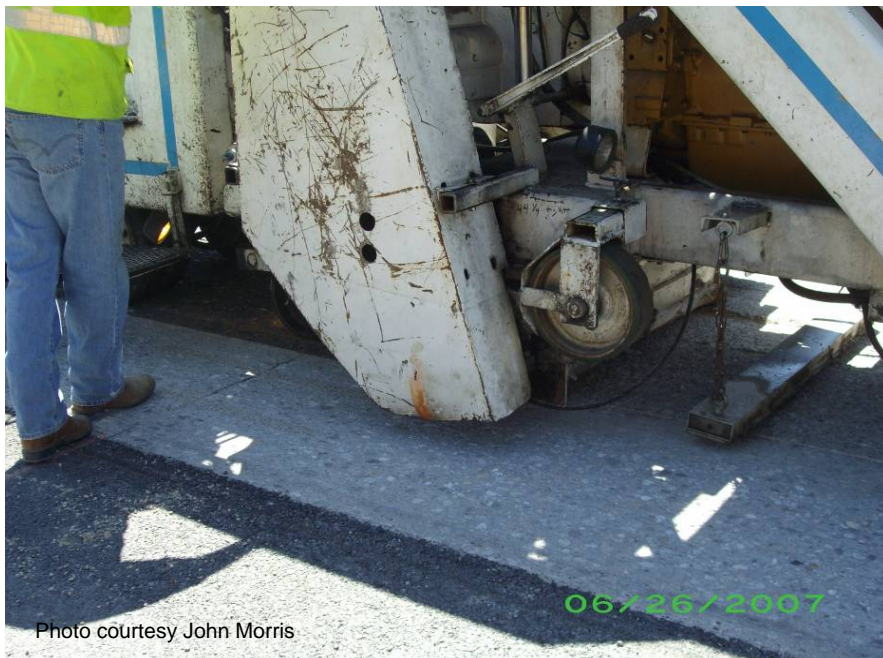
Figure 82 Diamond grinding equipment.
