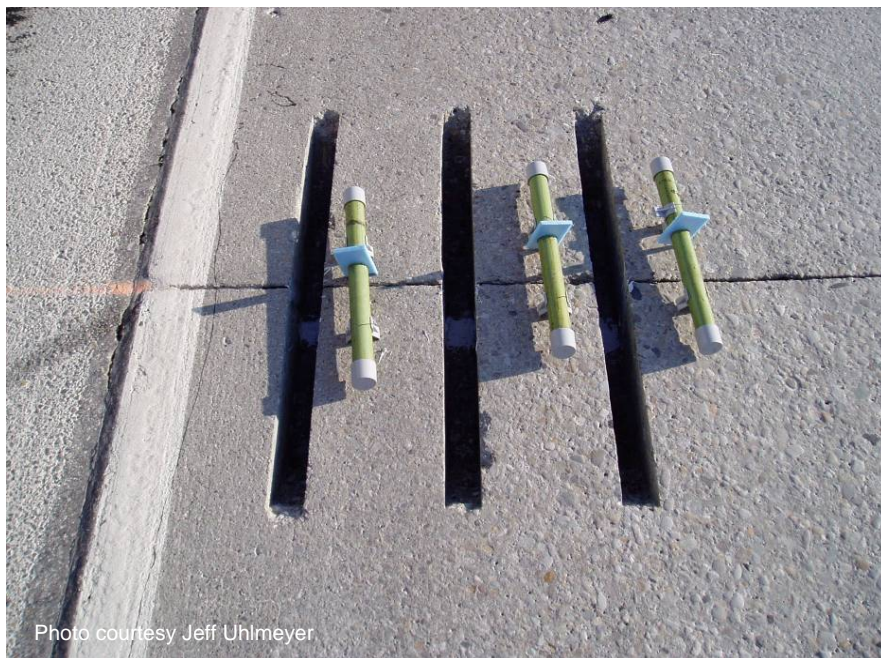
Figure 53 Close-up of dowel bar retrofit assemblies.
