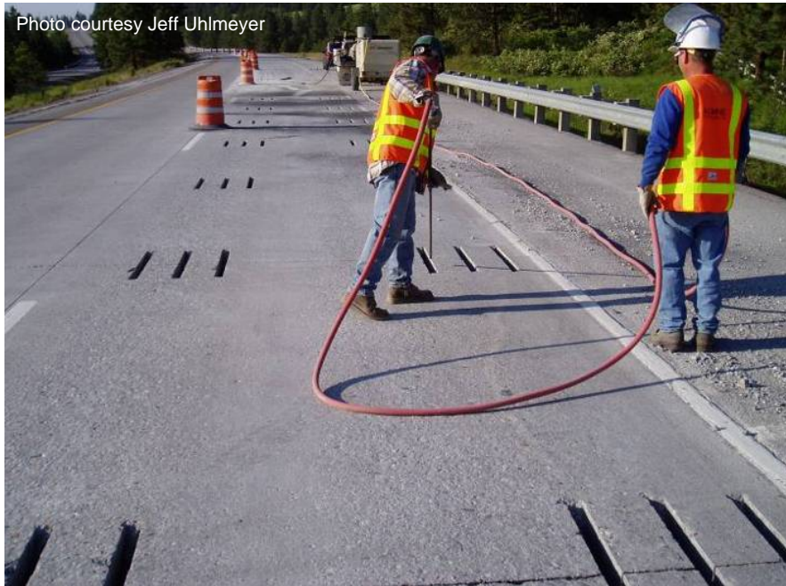
Figure 40 Cleaning dowel bar slots with compressed air.
