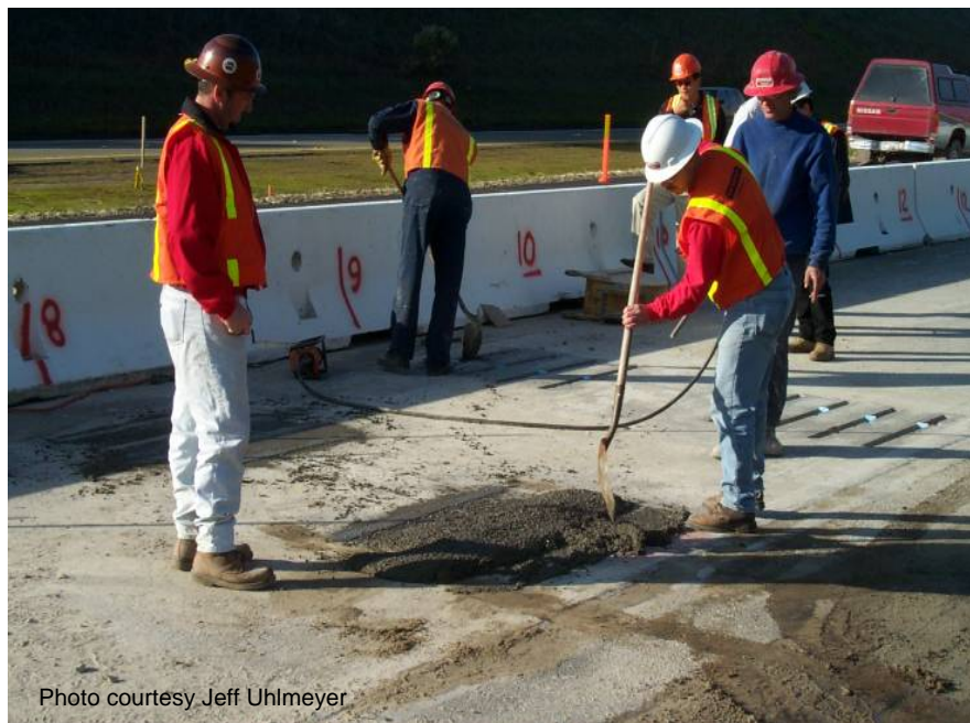
Figure 64 Moving patching material into dowel bar slots.
