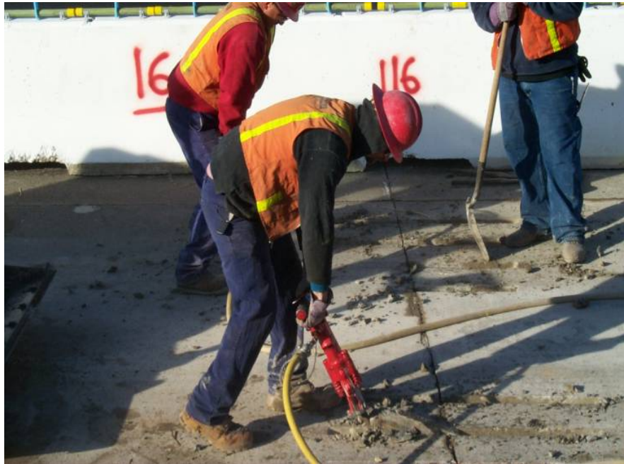
Figure 22 Maintain jackhammer at no more than a 45-degree angle.
