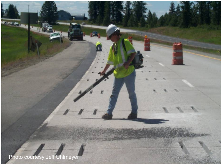
Figure 38 Cleaning shot blasting debris from roadway.
