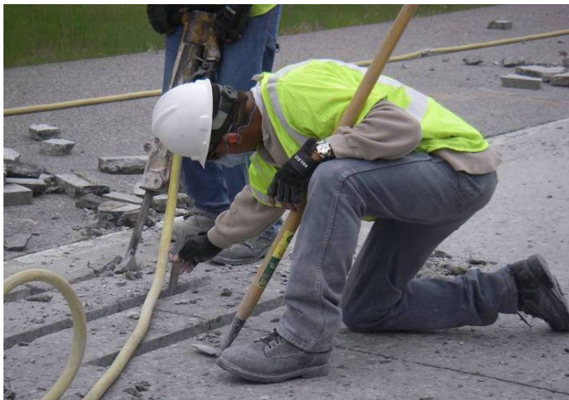
Figure 16 Check depth of dowel bar slot.
