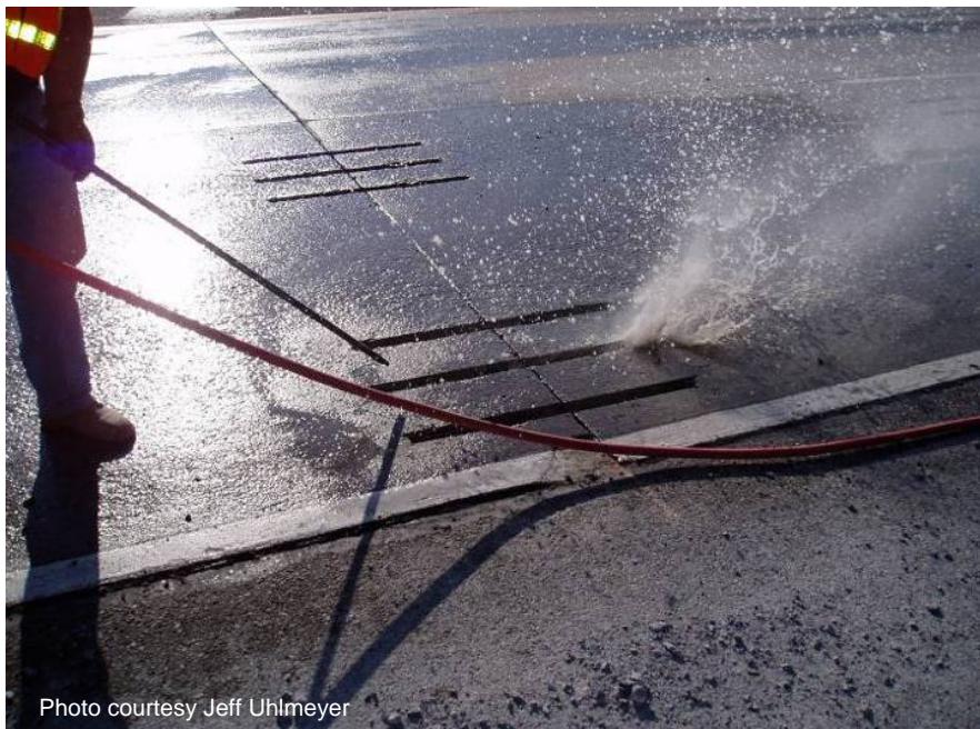
Figure 39 Removing water and other debris with compressed air.
