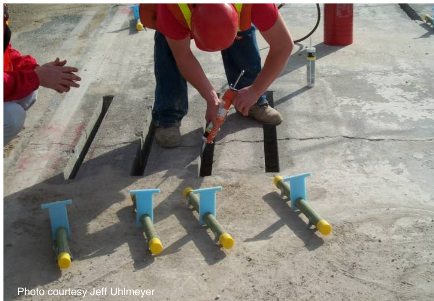
Figure 49 Caulking dowel bar slot sides and bottom.
