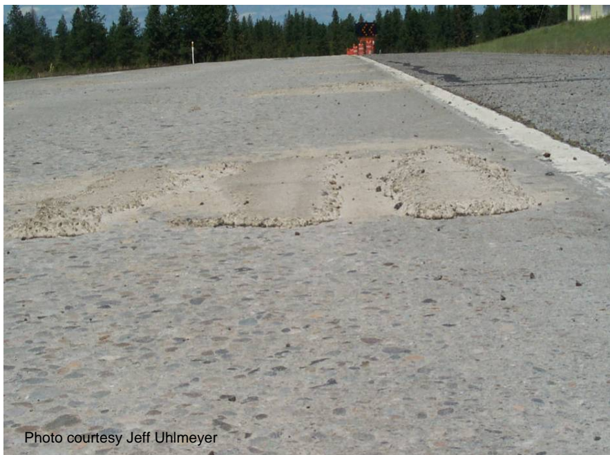
Figure 73 Patching material left high to minimize segregation.
