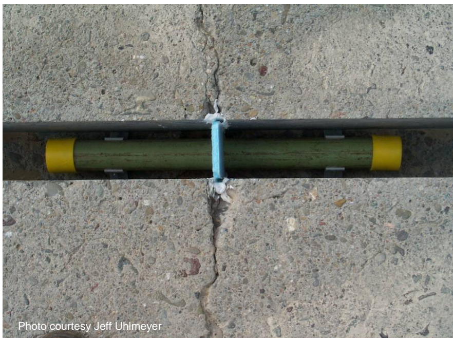
Figure 57 Close-up of dowel bar retrofit assembly at a transverse crack.
