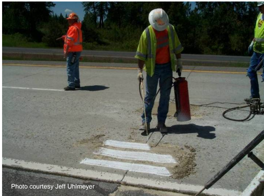
Figure 74 Applying curing compound.
