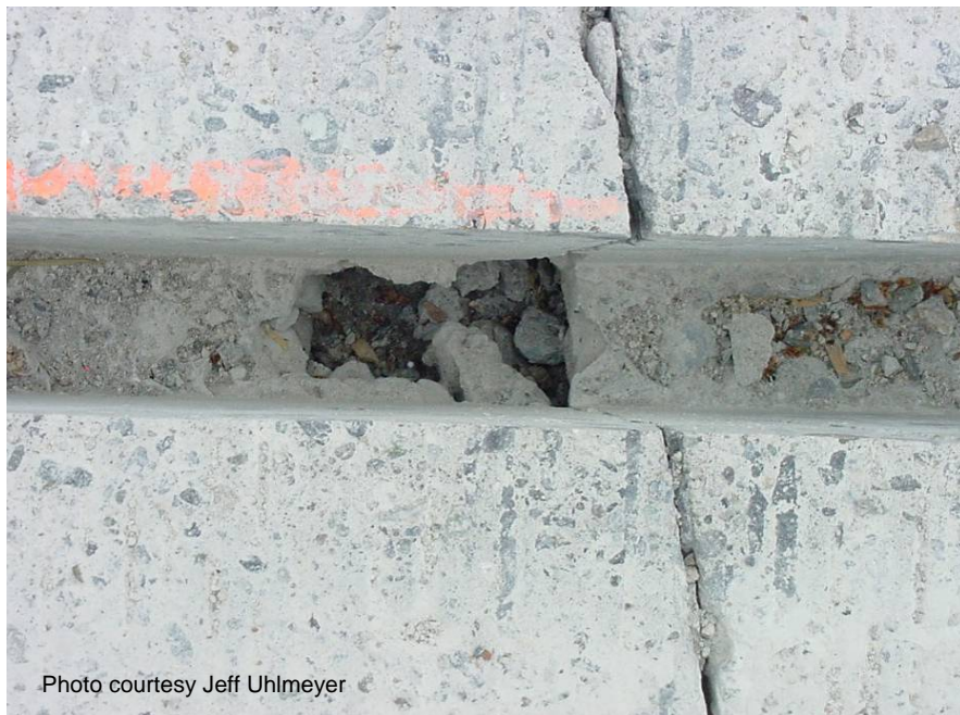
Figure 30 Jackhammer punching through the bottom of the dowel bar slot.
