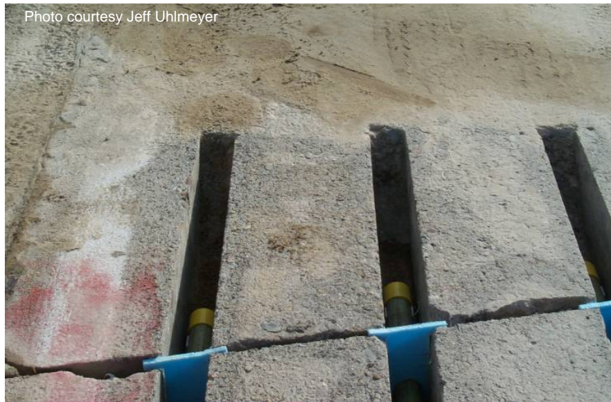
Figure 48 Debris should be cleared to a sufficient distance to prevent intrusion.
