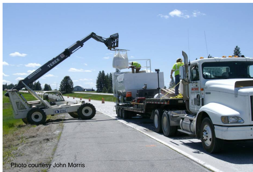
Figure 61 Delivery of materials to mobile mixer.
