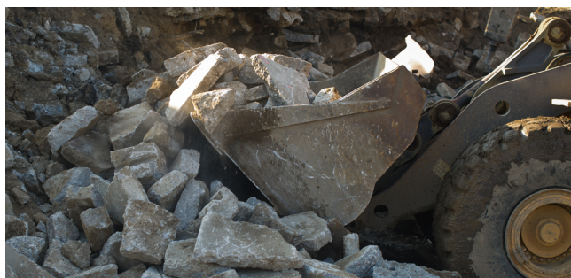
Figure 5-8. Concrete pavement for recycling (photo courtesy of Michigan State University)
