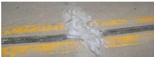
Figure 5-6. Pre-overlay repair of spalled joint (photo courtesy of Todd LaTorella, MO/KS ACPA)
