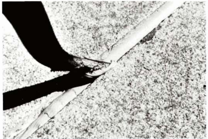
Figure 18 Close-up of low-modulus silicone sealant tooling.
